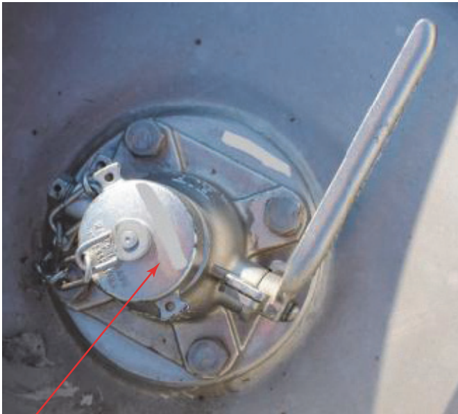
INLET VALVE AND CAP
