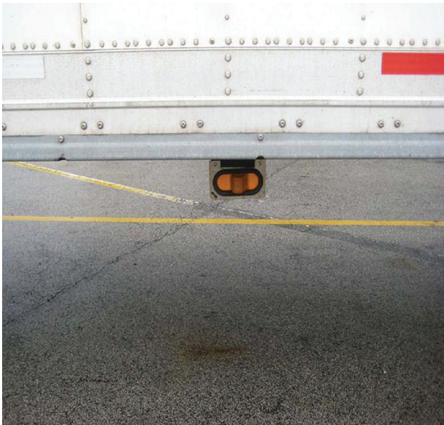
Fig. 6.1 Light correctly positioned away from lift points
