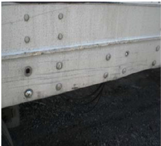
Fig. 2.10 Securement defect—missing rivets
