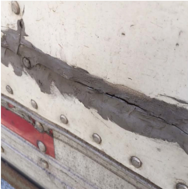
Fig. 2.27 Side panel breaks/cracks
