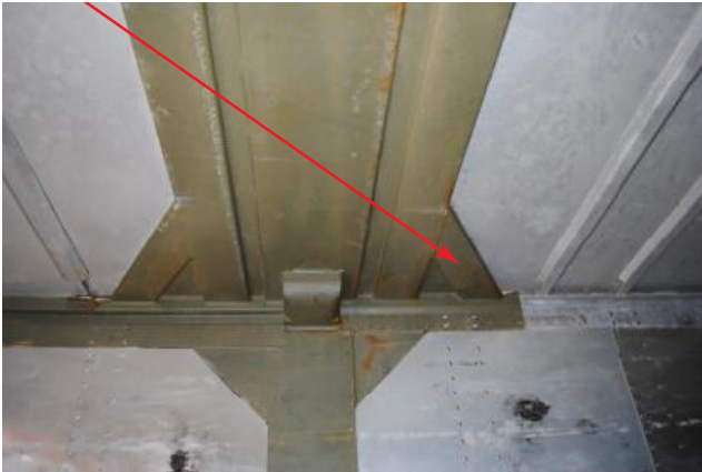
INTERMEDIATE HEADER GUSSET
