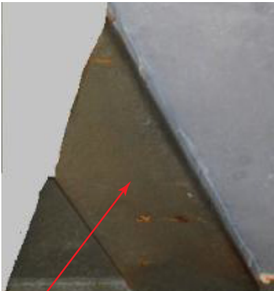
INTERMEDIATE HEADER GUSSET
